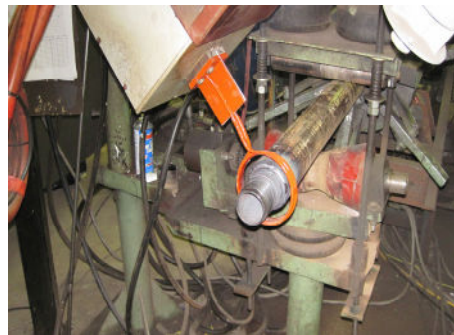
Post Weld Heat Treating
